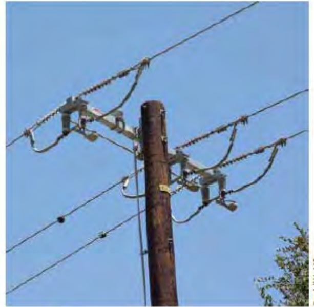
Figure 5.23 Disconnect switches.
