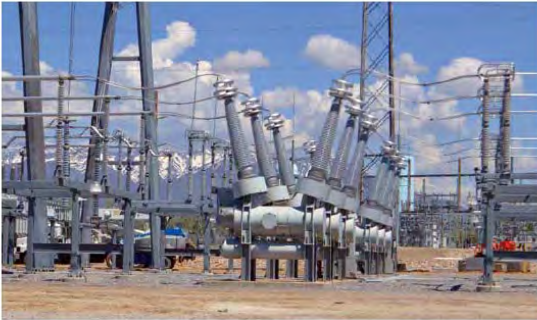
Figure 5.25 Circuit breakers.
