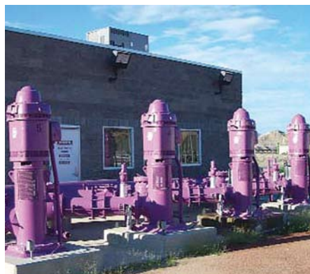
Purple pumps at this El Paso treatment plant are part of a system that reclaims wastewater for non-potable uses.
