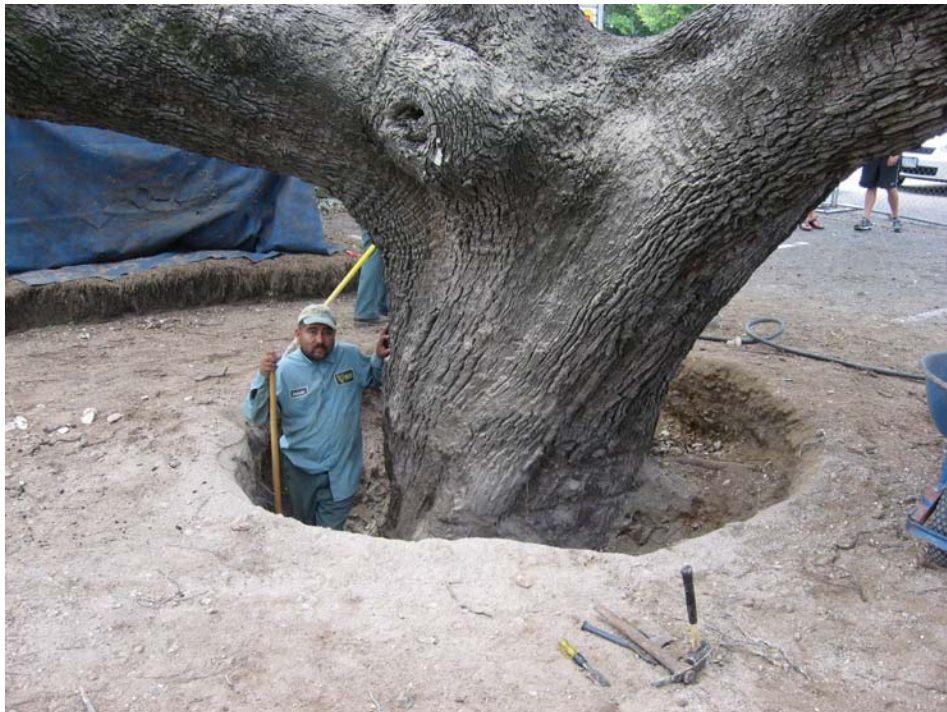
Image 3: Exploratory root collar excavation.
